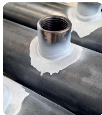
Liquid penetrant testing
