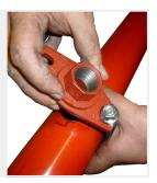
Tighten both nuts alternately with an impact wrench (with the appropriate cap) until they are firmly attached. You can then tighten the U-bolt to the specified torque using a torque wrench. (Applying a higher torque will not improve the sealing and may damage the piece). The sprinkler tee must be level.
