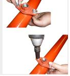
NOTE: For proper sealing, torque standards must be respected. A torque too big cannot improve the sealing property of the coupling, on the contrary, it will damage the bolts and housing, even cause disconnections. A torque too small will lead to leakage. Both disconnections and leakage may cause injuries or impairements to the installation.
